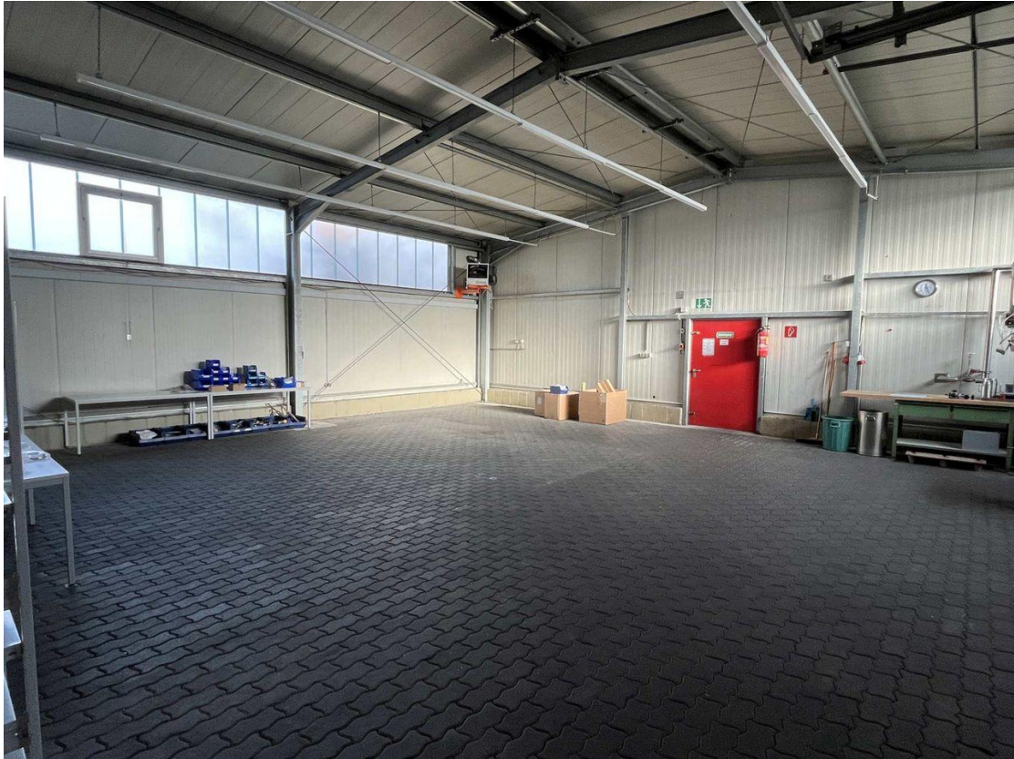
Blick in Halle I
